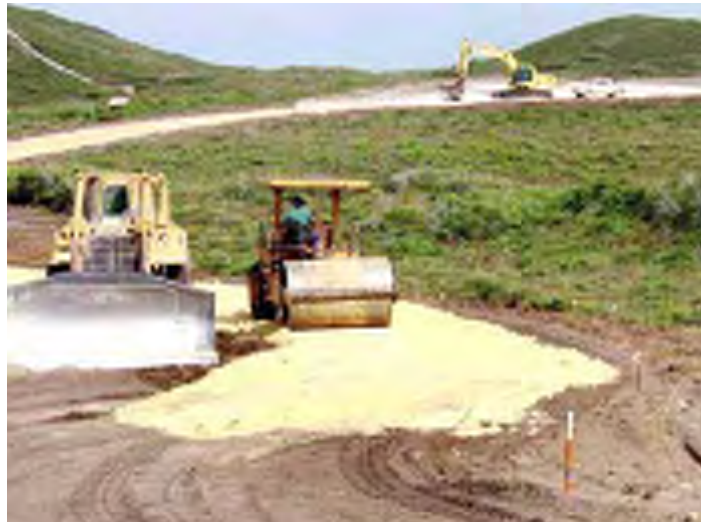
Figure 3 Typical Turbine Access Road under Construction
