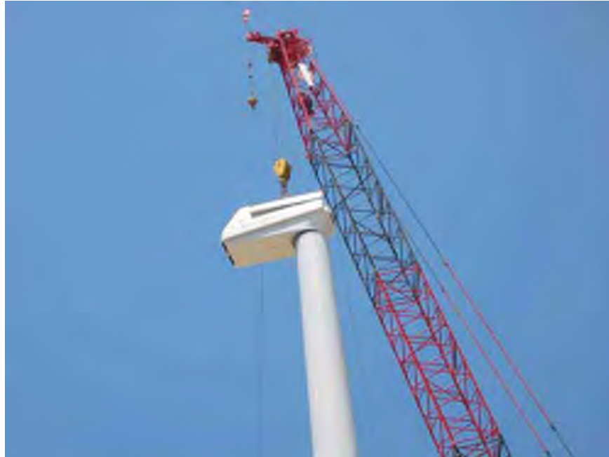
Figure 20 Nacelle Placement
