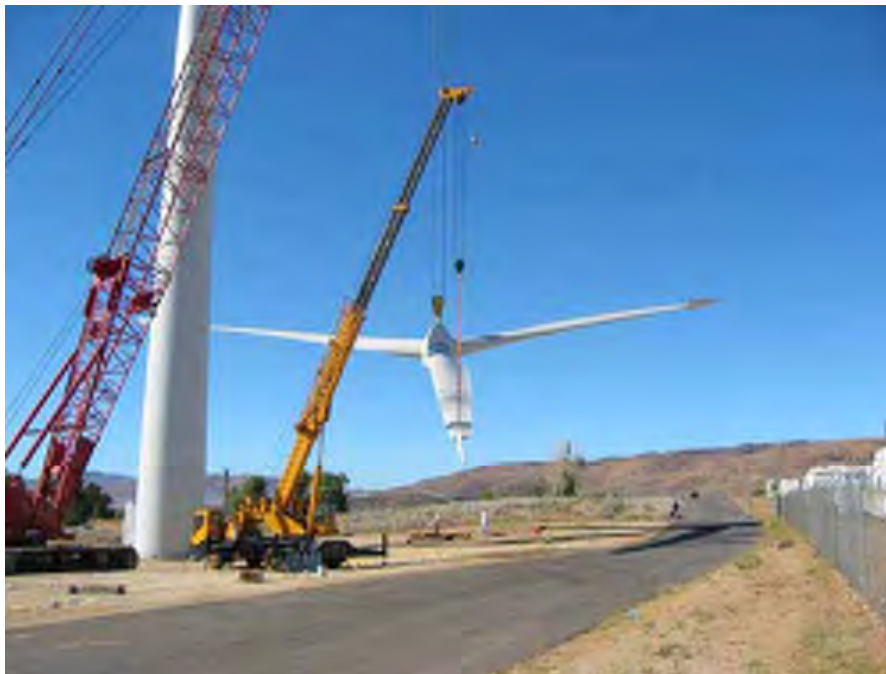
Figure 21 Complete Rotor Pick-Up
