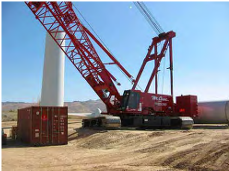
Figure 18 Tracked Crane on Crane Pad
