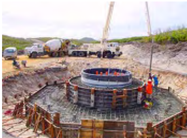
Figure 5 Mat Foundation Installation
