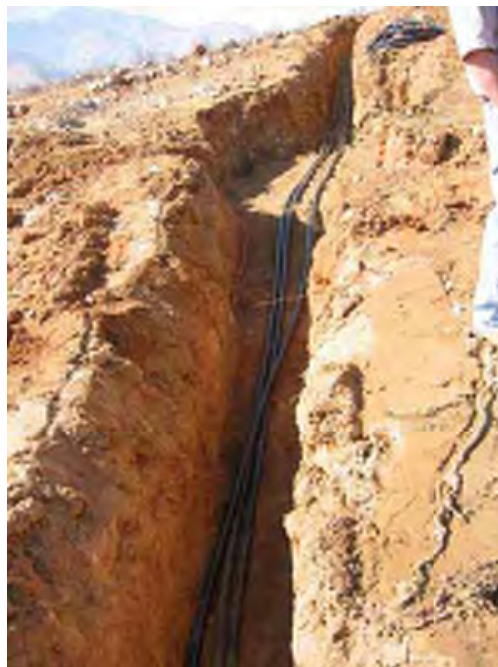
Figure 13 Open Trench Example
