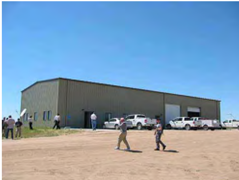
Figure 10 Typical Operations and Maintenance Building
