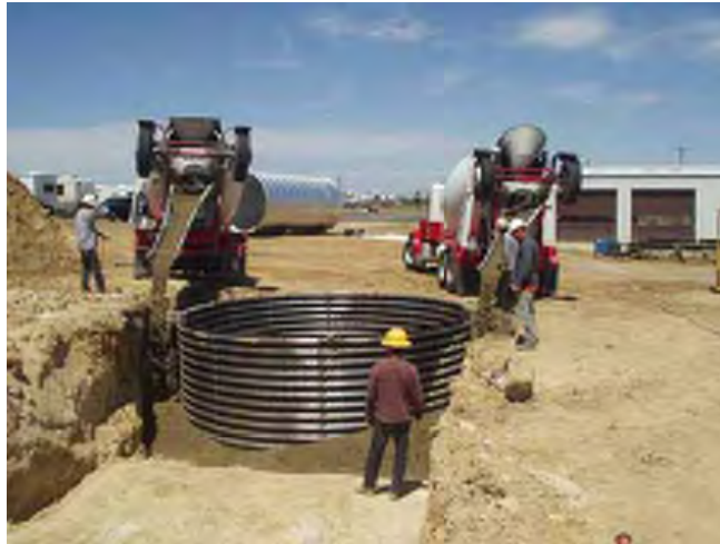
Figure 6 Pier Foundation Installation
