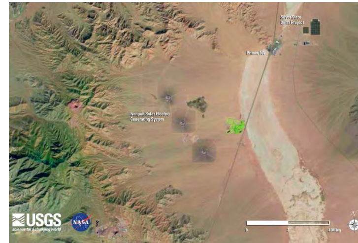
Ivanpah Solar Electric Generating System
