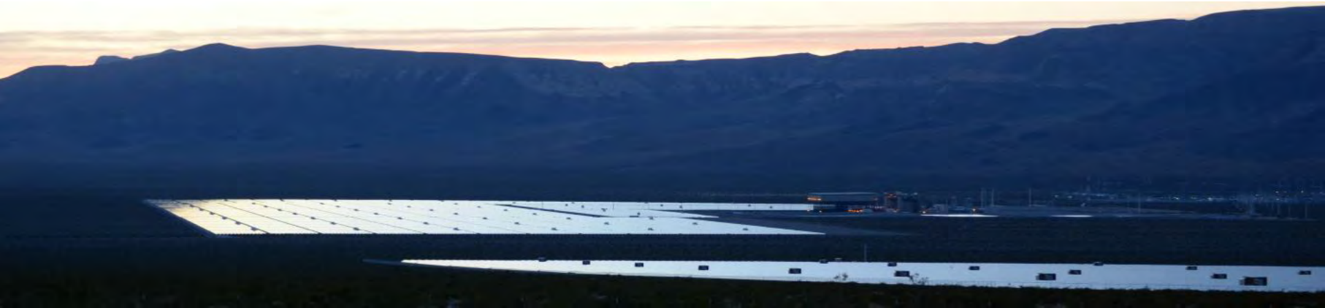
Copper Mountain PV facility in southern Nevada. Example for the “lake effect” hypothesis. Photo Credit: Robert Sullivan, Argonne National Laboratory
