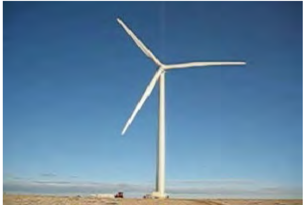
93-m diameter RSA and 2.5 MW
