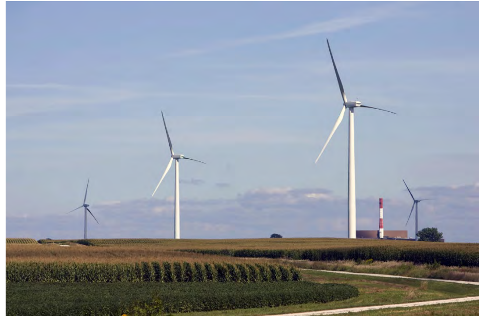
Grand Ridge Wind Energy Center. GE 1.5-MW turbines in LaSalle County, Illinois. Photo by Invenergy, LLC, NREL 16040.
