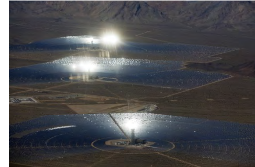
Ivanpah Solar Electric Generating System
